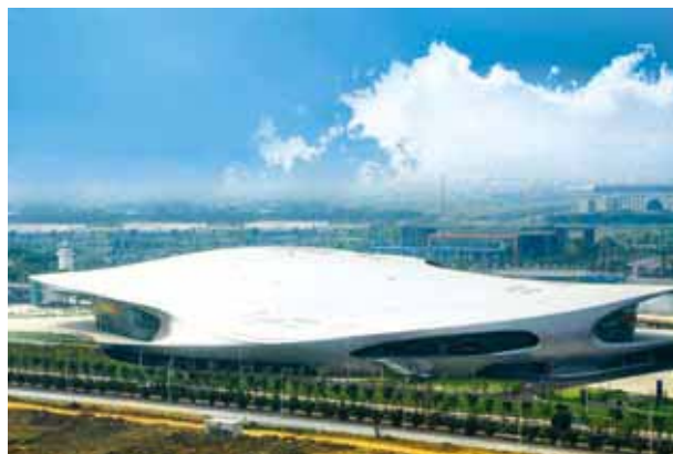
Guangzhou Asian Games Town Gymnasium metal roof construction project
