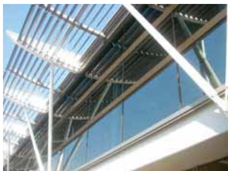
Curtain Wall System for the North Satellite Concourse Building at Hong Kong International Airport
